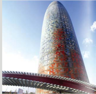
Torre Agbar, Barcelona, Spain
